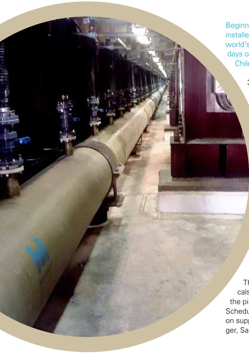
Beginning of December 2011, 18 workers from HOBAS Kunststofftechnik installed roughly 800 meters of HOBAS GRP Pipe with CPVC liner in the world's biggest copper mine. The line has been completed within four days only and under extremely challenging working conditions in the Chilean Atacama desert 3200 m above sea level.
